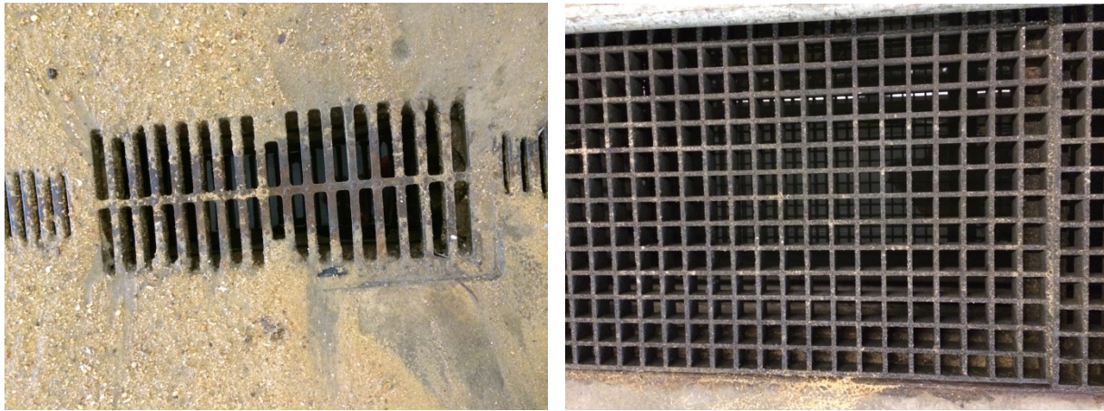
Figure 85. Catch Drain in the Water Reclamation System
