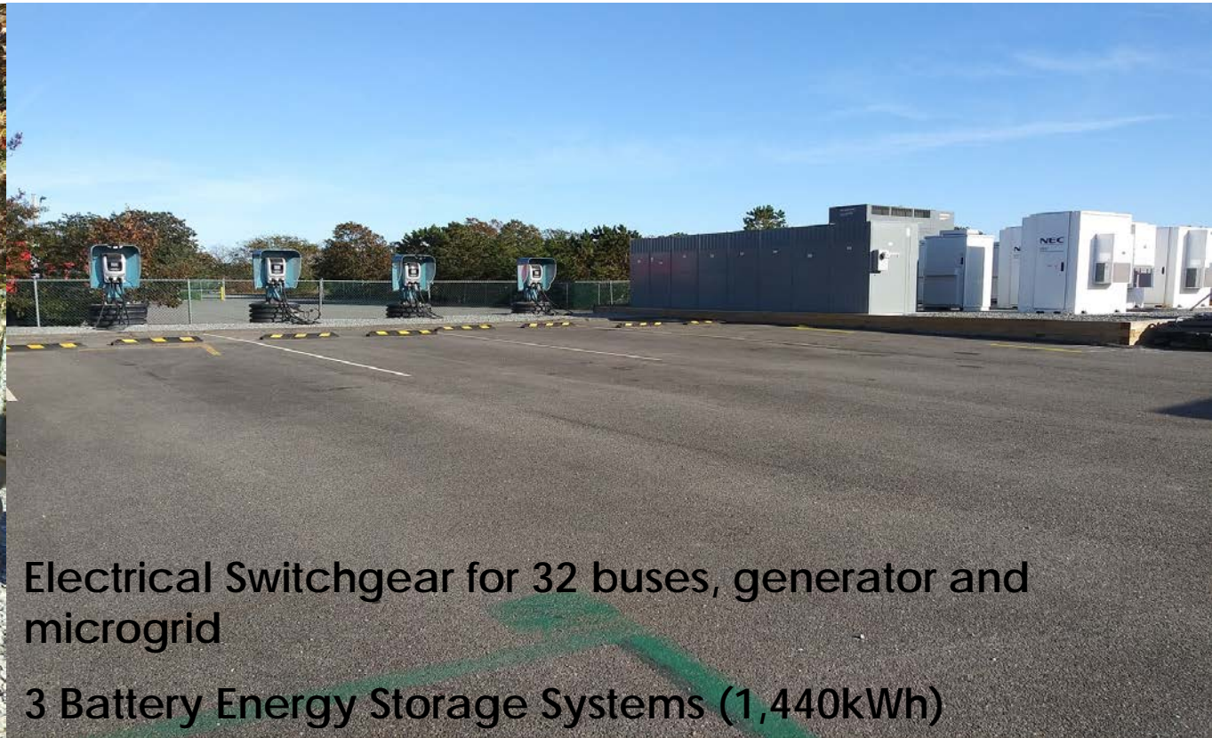
12 – 80kW Bus Chargers Installed, bases for 14 more are already installed
